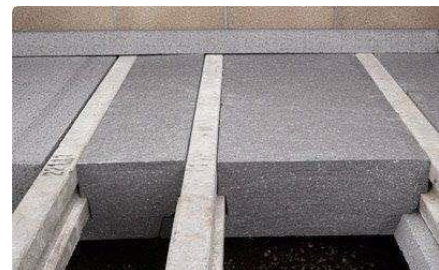
Figure 6. Slab filling polystyrene with concrete (Source: konnyu-beton.hu)
