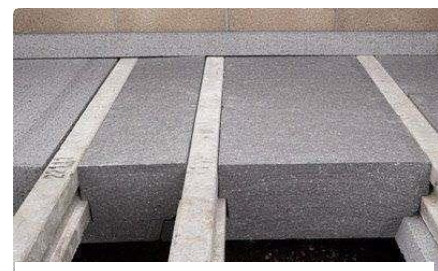
Figure 6. Slab filling polystyrene with concrete (Source: konnyu-beton.hu)
